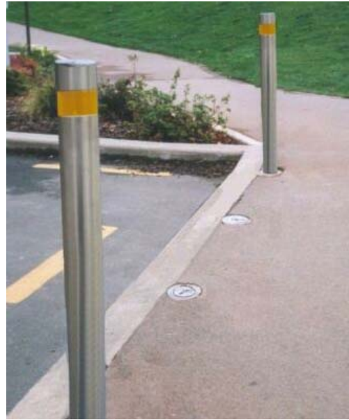
Retractable Bollards provide access in high use areas.
